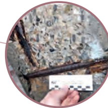
Modernised section 16, motorway overpass EXIT 119 Velký Beranov, registration No DN1-161.1
