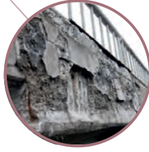
Modernised section 02, motorway bridge EXIT 21 Mirošovice, registration No D1-30.1
